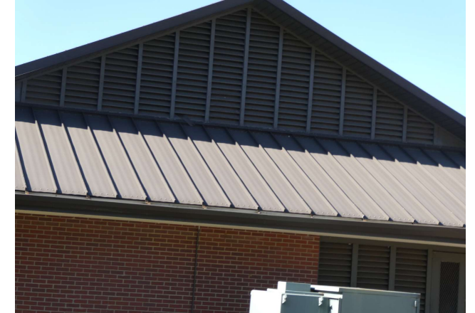
Typical metal roof at the kitchen/cafeteria building.
