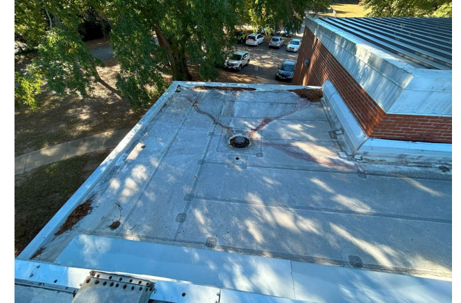
Overview of TPO roof covering.
