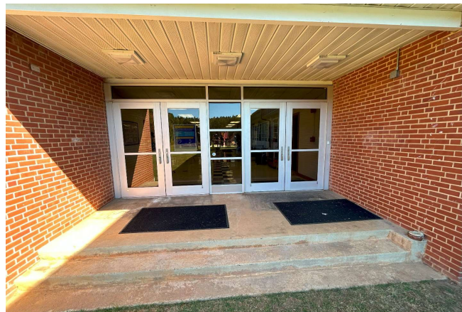
Storefront systems are in good condition.
