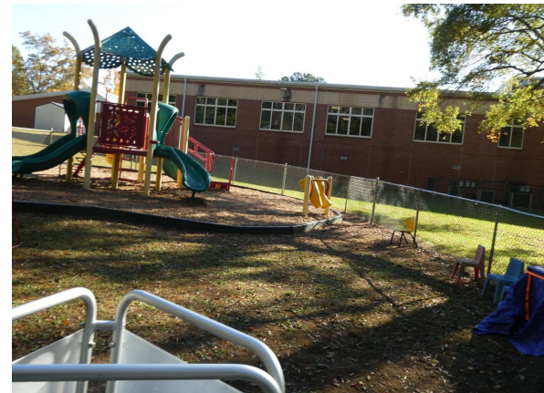
Playground and exterior façade on west side
